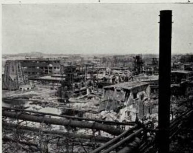
Photo 57. The Fischer-Tropsch catalyst manufacturing plant. This is a general view looking east at the catalyst plant known as Kartor-Fabrik-Lutzkendorf. ✓
