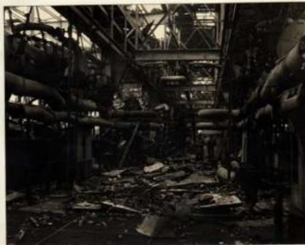
Photo No. 68. F-T CONTACT OVEN HOUSE. (Plot Plan No. 641). (Middle pressure) General view of damage down the control aisle.
