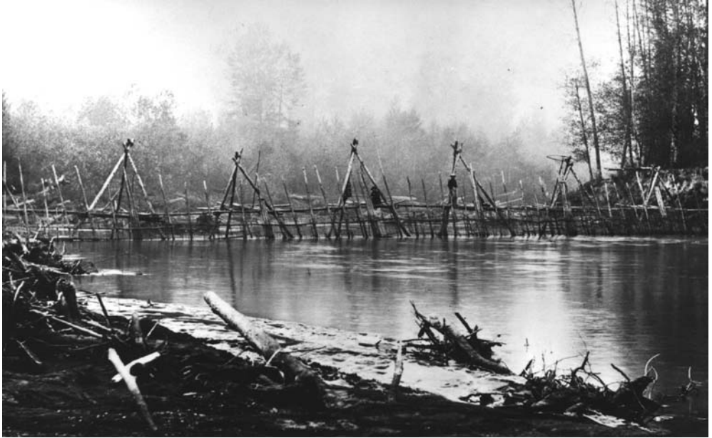
Chehalis Indians fishing on the Chehalis River, ca. 1900. Chalcraft explained in his memoir that elaborate platforms were built across the Chehalis River and wooden spears (in plentiful runs even pitchforks) were used for killing and securing the fish. (photo courtesy of Hazel Pete Family)
