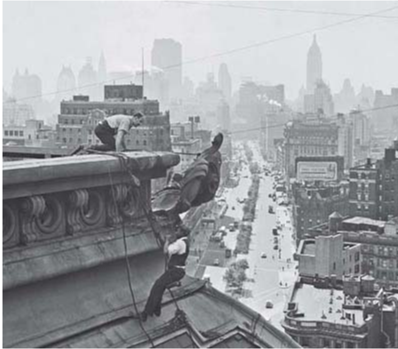
NOTHING WAS OVERLOOKED during the city's scrap metal drive. Here, workers remove one of four 100-pound cornices on the roof of the Ansonia Hotel at Broadway and 73rd Street. Thousands of pounds of metal would be gathered from the hotel roof's ornamentation. AP Images.
