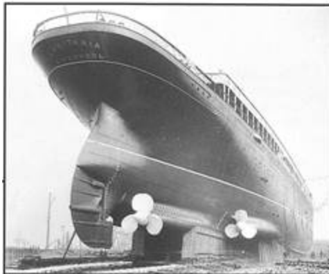
Stern view of the Lusitania under construction in the yards of John Brown on the Clyde, 1905.
