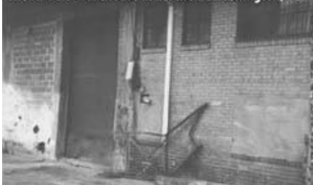
The Finders' warehouse in northeast Washington, DC.
