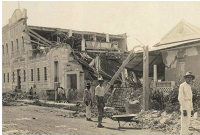
Figure 39. Photo of 1918 earthquake damage in the Puerto Rico city of Mayaguez. Source: Wikimedia Commons, University of Puerto Rico (photo, Cifuentes).
